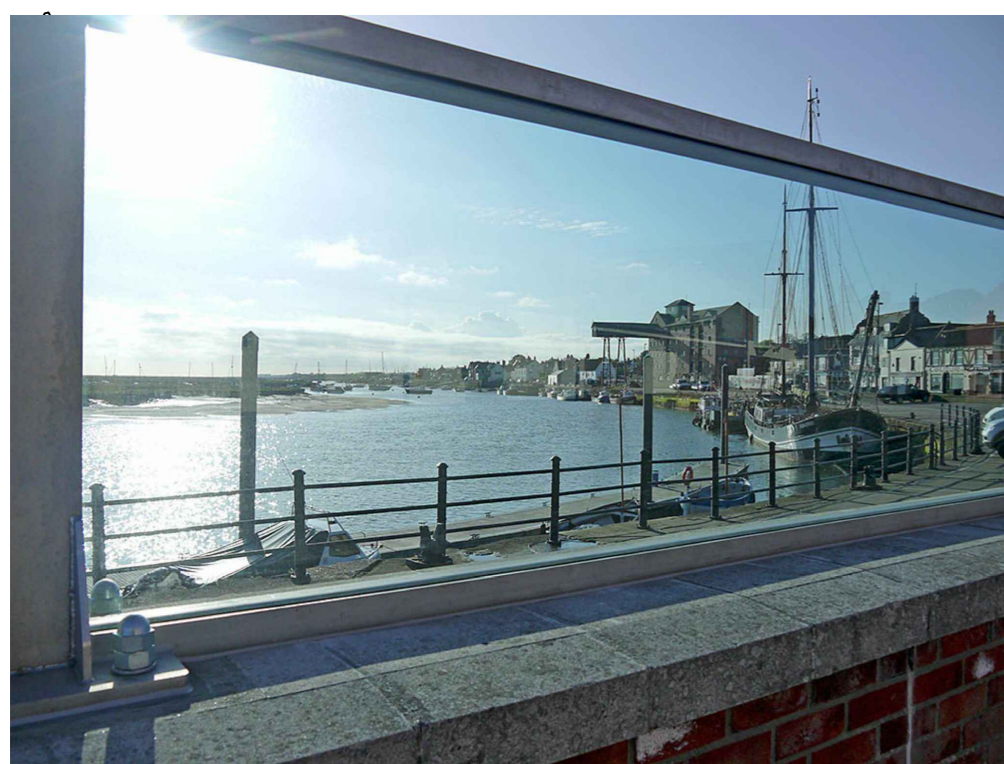
Example of glass flood defence panels
